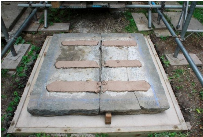
The bottom bed of the moulded plinth (to be applied) had been worked flat so a uniform coarse mortar bed was applied, to allow the endless slings to be removed without fouling the mortar. Note the blue chalk lines denote exactly where the plinth is to be placed.
