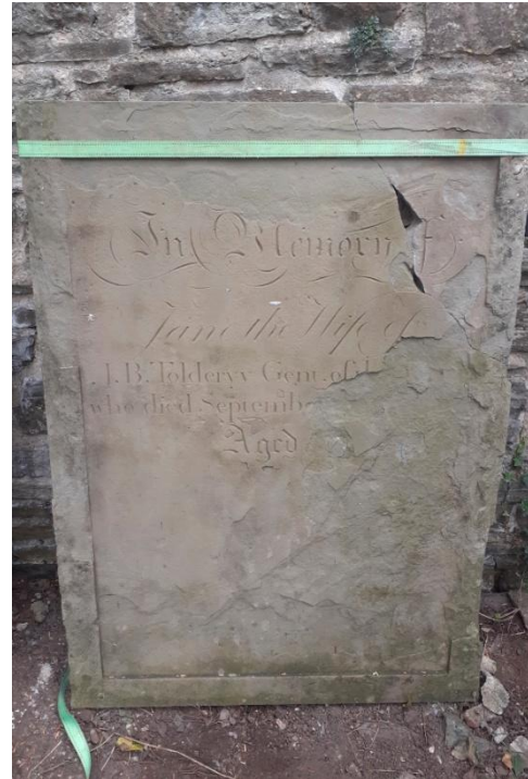
The front inscription before and after re-joining broken sections. Resin was kept well-back from the front face so it was not visible and the effected joins look as 'natural' as possible. Note the loss of detail to both vertical, raised borders and the bottom right-hand corner, much of the carved upper surface has been lost from this very laminar stone type.
