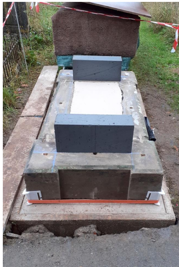
On the left the new re-enforced sub-base in position with the plinth blocks having been bedded into position. On the right, the void within the plinth has been filled with Limecrete, on top of a Visqueen DPM/separation layer. Celcon blocks being laid to create a supporting internal core.
