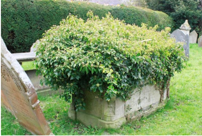
The tomb chest before any treatments, highlighting the extent of well-established ivy growth, which disguises the extent of structural damage to the memorial.
