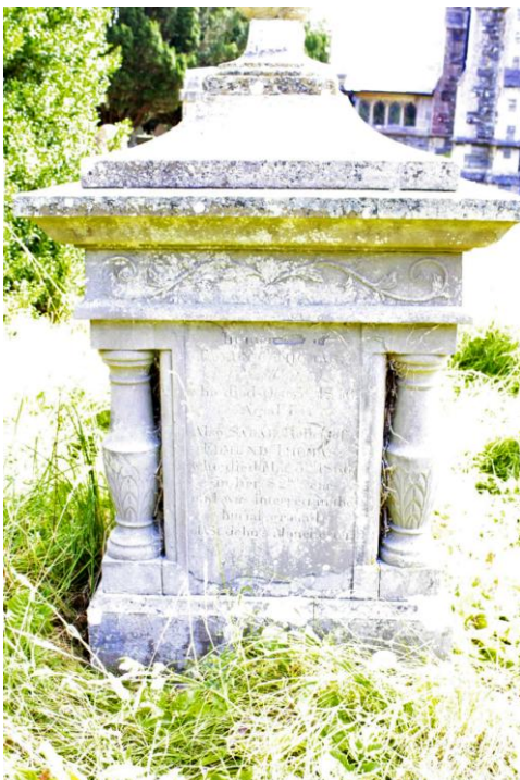
The west elevation of the Thomas memorial before and after all treatments. Delaminated stone along the bottom bed of this elevation was also rationalised back to sound substrate, with support fillings inserted along the length of the previously tacked edges. Carved detail to the frieze is a little easier to determine on this elevation.
