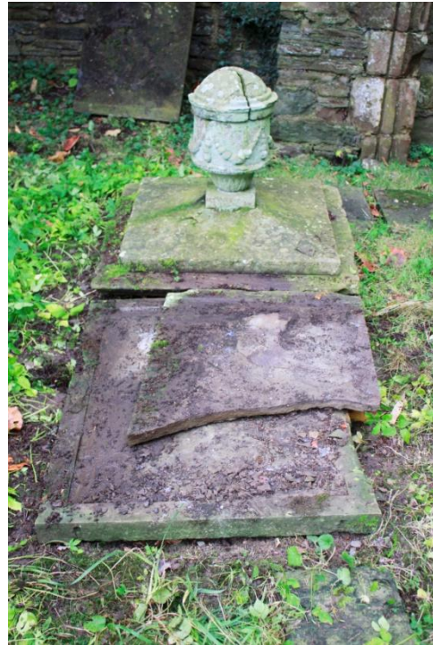
The box-tomb elements stacked haphazardly on top of each other with several of the side panels having fractured as a result of point-loading from uneven weight distribution. Note the extent of soil and debris on the upper surfaces and fractures through the urn-lid clearly visible.
