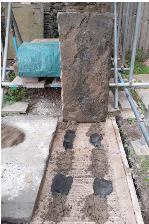
The newly joined section before bedding on mortar and slate packers. The whole perimeter was deep-tamped with mortar. Once this had hardened sufficiently liquid grout (based on NHL3.5) was introduced into the join from front to back, to provide additional support once hardened.
