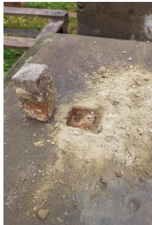
Iron cramps in the top-bed of the tomb chest secured with sound, lime-mortar and square-section studs in the bottom bed of the tomb chest, which weren't replaced. The studs prevented even more movement in the subsiding memorial. These weren't replaced as the memorial will be stable on its new re-enforced concrete sub-base.
