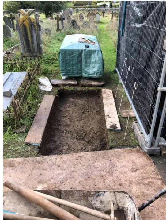
On the left the plinth showing how much subsidence has taken place and how much the churchyard has risen over the 186 years since it was likely built. On the right, the plinth blocks have been moved. There were only two re-cycled tomb chest slabs at the far, east end, providing any sort of sub-base. Note the proximity of the railings and underlying kerb-set to the north.
