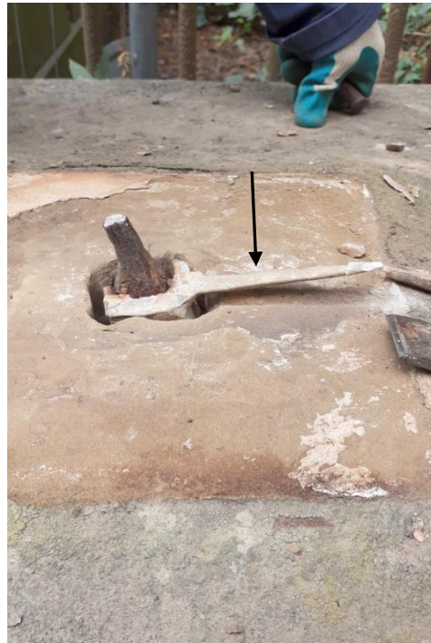
Drilling around the lead 'encased' iron-dowel to release it, which was completely ineffective and didn't prevent delamination of the ferrous metal. Note the route of the molten lead (indicated) introduced into an oversize vertical hole, but ineffective once excess moisture gets into the joint, when pointing fails. Original holes were re-used where appropriate, often needing to make them deeper, to accommodate longer stainless-steel dowels which will not corrode.
