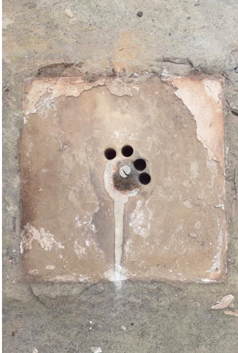
Drilling around the lead 'encased' iron-dowel to release it, which was completely ineffective and didn't prevent delamination of the ferrous metal. Note the route of the molten lead (indicated) introduced into an oversize vertical hole, but ineffective once excess moisture gets into the joint, when pointing fails. Original holes were re-used where appropriate, often needing to make them deeper, to accommodate longer stainless-steel dowels which will not corrode.
