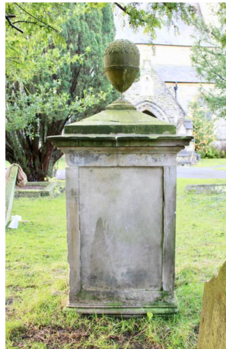
The rear, north elevation before (left) and after all treatments. Note how the moulded entablature (indicated) shows a dovetailed, vertical, central-joint, due to failed fixings - causing point-loading on the 'short' box panels beneath, at the front and back. That situation was significant on this elevation, contributing to the inside of the panel delaminating in half and being substantially weaker as a result. The resultant joints lines have all been pointed from back to front, with a fluid, gunnable mortar.
