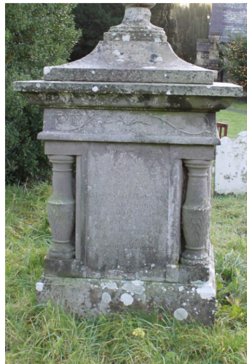
The west elevation of the Thomas memorial before and after all treatments. Delaminated stone along the bottom bed of this elevation was also rationalised back to sound substrate, with support fillings inserted along the length of the previously tacked edges. Carved detail to the frieze is a little easier to determine on this elevation.
