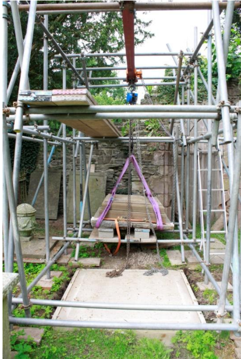
Once the concrete padstone had reached compressive-strength, the sub-base and plinth were moved horizontally and lowered into position. Unfortunately whilst lowering the 'whole', the right-hand half of the sub-base fractured and detached from the moulded plinth, with only mortar between the two courses and no fixings.
