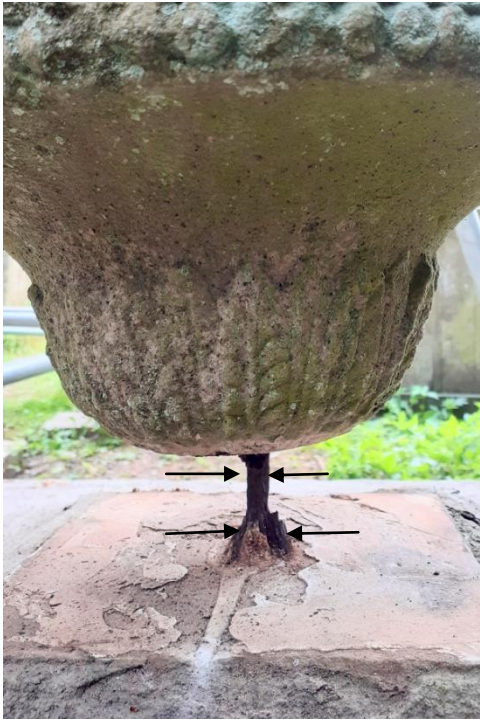
The expanded dowel spanning vertically between the capstone and the bottom bed of the It had split the thin base into four sections but luckily not disrupted the capstone. Note the actual size of the original dowel, which was secured with molten lead and the expanded size of the corroded metal (both indicated).
