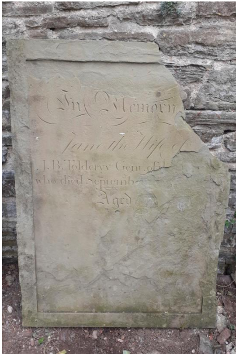
The front inscription before and after re-joining broken sections. Resin was kept well-back from the front face so it was not visible and the effected joins look as 'natural' as possible. Note the loss of detail to both vertical, raised borders and the bottom right-hand corner, much of the carved upper surface has been lost from this very laminar stone type.
