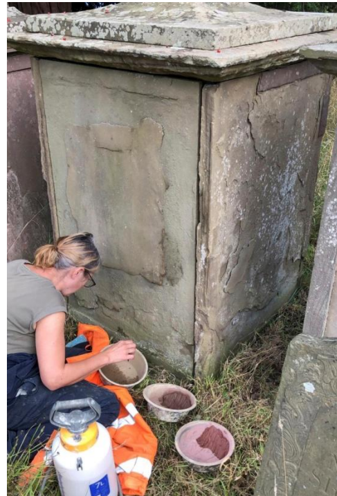
On the left, the south elevation highlighting the simple border in the foreground (indicated) has delaminated and detached from this 'long' side. This side was rationalised hard prior to inserting support fillings. On the right, support fillings being inserted into vulnerable edges, before the capstone is removed/replaced. Note the plinth is not visible on these two elevations with ground level having risen to cover it.
