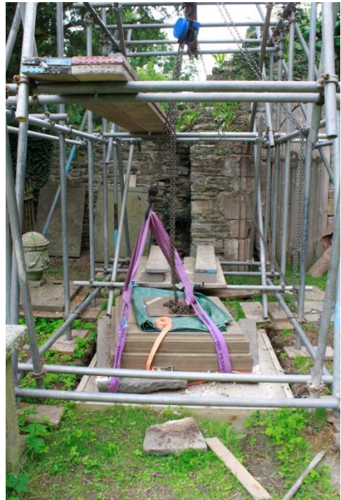
Once the concrete padstone had reached compressive-strength, the sub-base and plinth were moved horizontally and lowered into position. Unfortunately whilst lowering the 'whole', the right-hand half of the sub-base fractured and detached from the moulded plinth, with only mortar between the two courses and no fixings.
