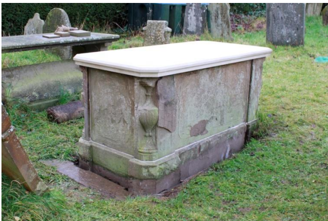
The tomb chest after all treatments, note the colour of the lid is because the stone is bone-dry, having been under-cover for many weeks. The three small, square, stone samples on the lid of the memorial in the background, is the true colour of the lid, with the samples having been outside for weeks.
