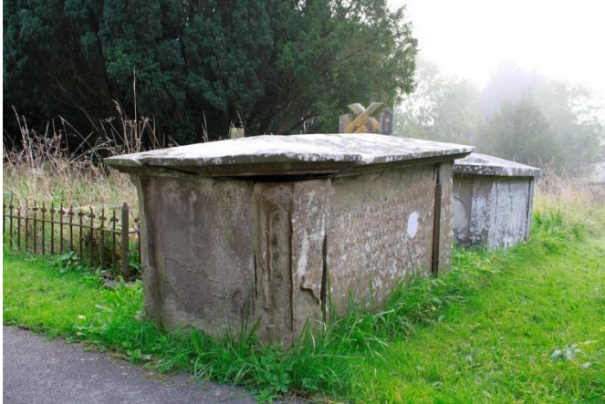
The memorial to William Powell before any treatments. Note the plinths proximity to the path, the degree of subsidence in the foreground, disruption/misalignment of the lid corner and delamination in the pilaster beneath that corner.
