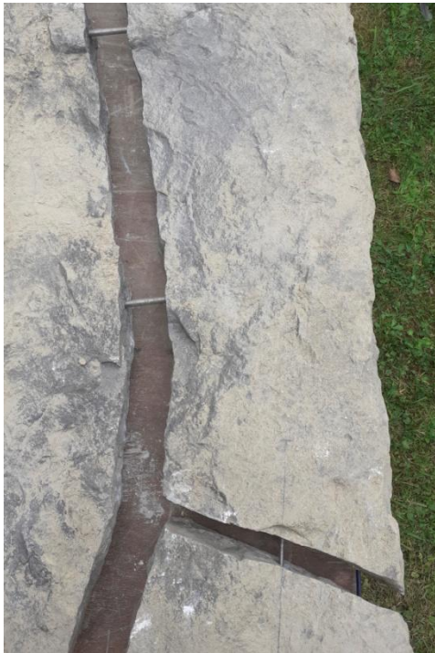
Three 12mm diameter, threaded stainless-steel dowels secured with epoxy-resin were employed to join the three sections as well as spots of resin on the mating break edges.
