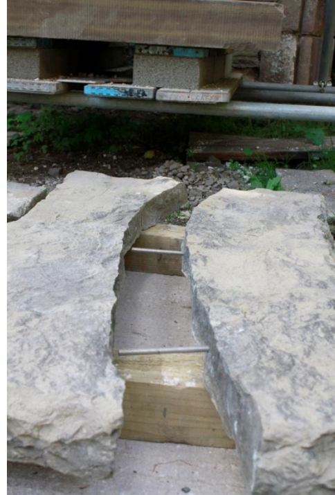
Three 12mm diameter, threaded stainless-steel dowels secured with epoxy-resin were employed to join the three sections as well as spots of resin on the mating break edges.
