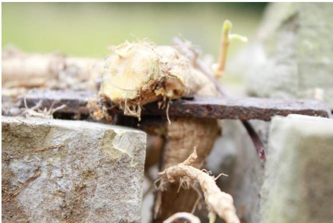
The ivy roots had forced apart many large, heavy sections but kept this dog-cramp (double turn-down) in place, by growth around it. The thick stems had forced these large stone blocks apart horizontally.
