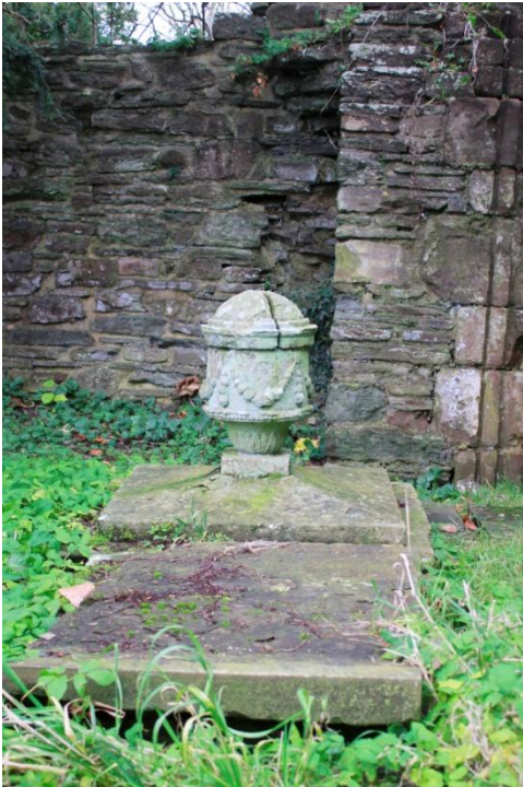
The box-tomb elements stacked haphazardly on top of each other with several of the side panels having fractured as a result of point-loading from uneven weight distribution. Note the extent of soil and debris on the upper surfaces and fractures through the urn-lid clearly visible.
