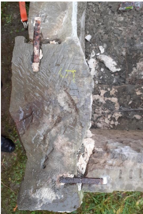
Iron cramps in the top-bed of the tomb chest secured with sound, lime-mortar and square-section studs in the bottom bed of the tomb chest, which weren't replaced. The studs prevented even more movement in the subsiding memorial. These weren't replaced as the memorial will be stable on its new re-enforced concrete sub-base.
