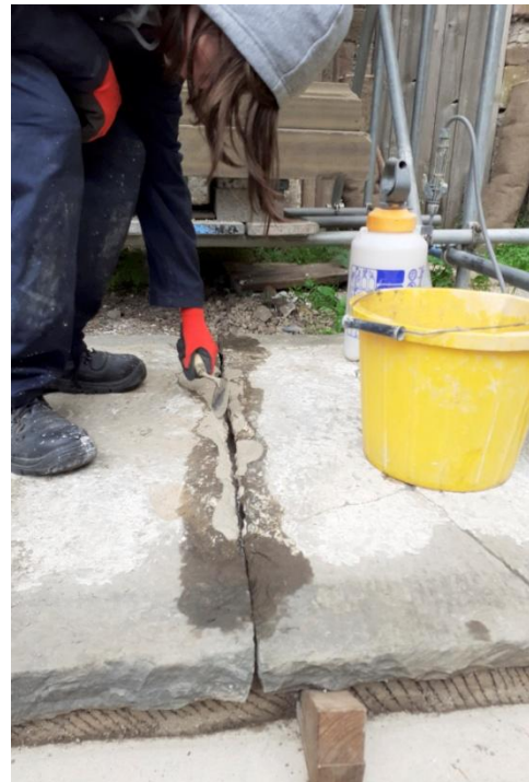
The newly joined section before bedding on mortar and slate packers. The whole perimeter was deep-tamped with mortar. Once this had hardened sufficiently liquid grout (based on NHL3.5) was introduced into the join from front to back, to provide additional support once hardened.
